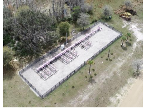
The manifold at the 4G Ranch Wetlands provides remote and automatic control with the ability to adjust cell water levels and flowrates and was constructed for easy access of equipment for maintenance.
