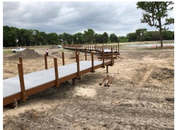
The boardwalks at The Ocala Wetland Recharge Park are a novel product consisting of a fiberglass pilings and framing and composite decking, providing a long-lasting product that requires little to no maintenance.
