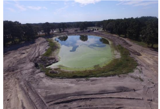
The design of the Ocala Wetland Recharge Park took advantage of existing ponds to provide open water habitats on the downstream ends of each wetland cells.
