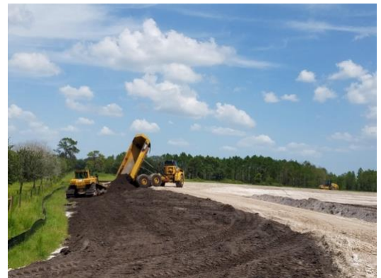
Effective stockpiling and re-spreading of topsoil from the site was used during the construction of the 4G Ranch Wetlands to support establishment of erosion protection grasses.
